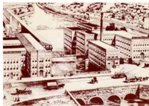
New Home Factory, Orange, MA
